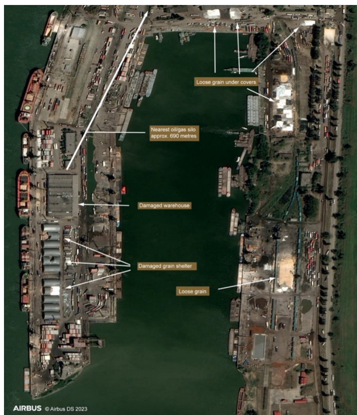
Figure 8: Satellite imagery dated 28 July 2023 showing the southern area of the port of Reni. Three shelters and a warehouse have been damaged with the nearest oil or gas silo being approximately 690 metres away. Grain is also in open storage under makeshift covers. © Airbus DS (2023) (annotated by GRC).
